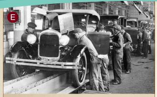
Henry Ford installed the first moving assembly line for the mass production of an automobile. He wanted to reduce the cost of car production so that almost everyone could have one. This innovation cut the build time from more than twelve hours to two hours and thirty minutes. When did this happen?
